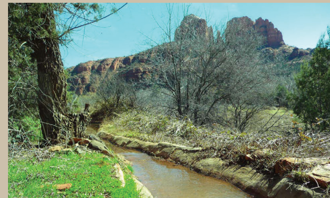
By the mid-1900s, the Dumas Ditch became clogged and cracked from neglect. The U.S. Forest Service cleaned and repaired it in the 1980s, enabling water to flow through this historic canal once again.
