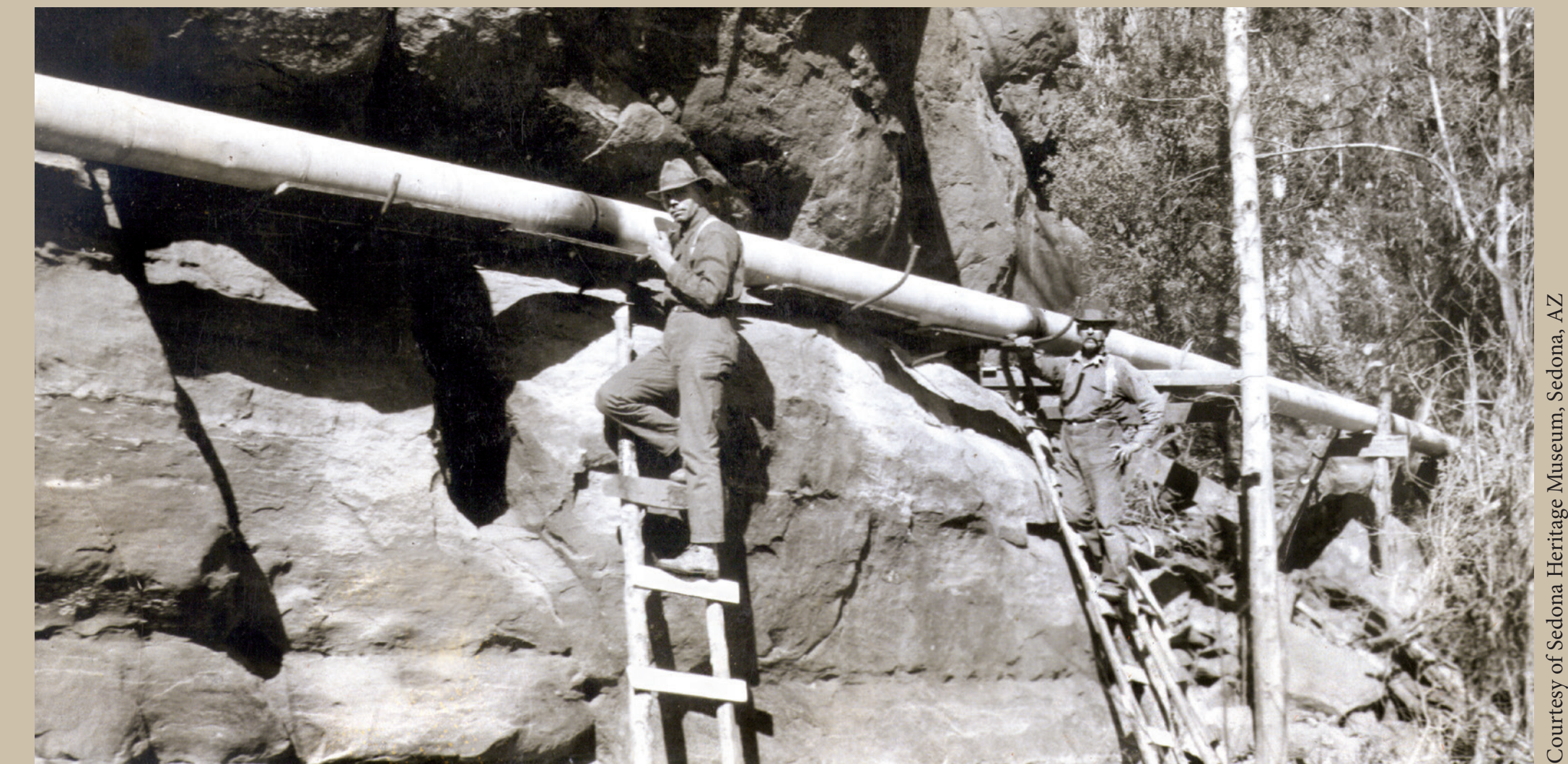
The Dumas and Schuerman families worked together in the early 1900s to construct an elaborate irrigation system on their ranch. Erwin Schuerman (left) repairs a section of the 1,500 feet of galvanized pipe used in the system.
