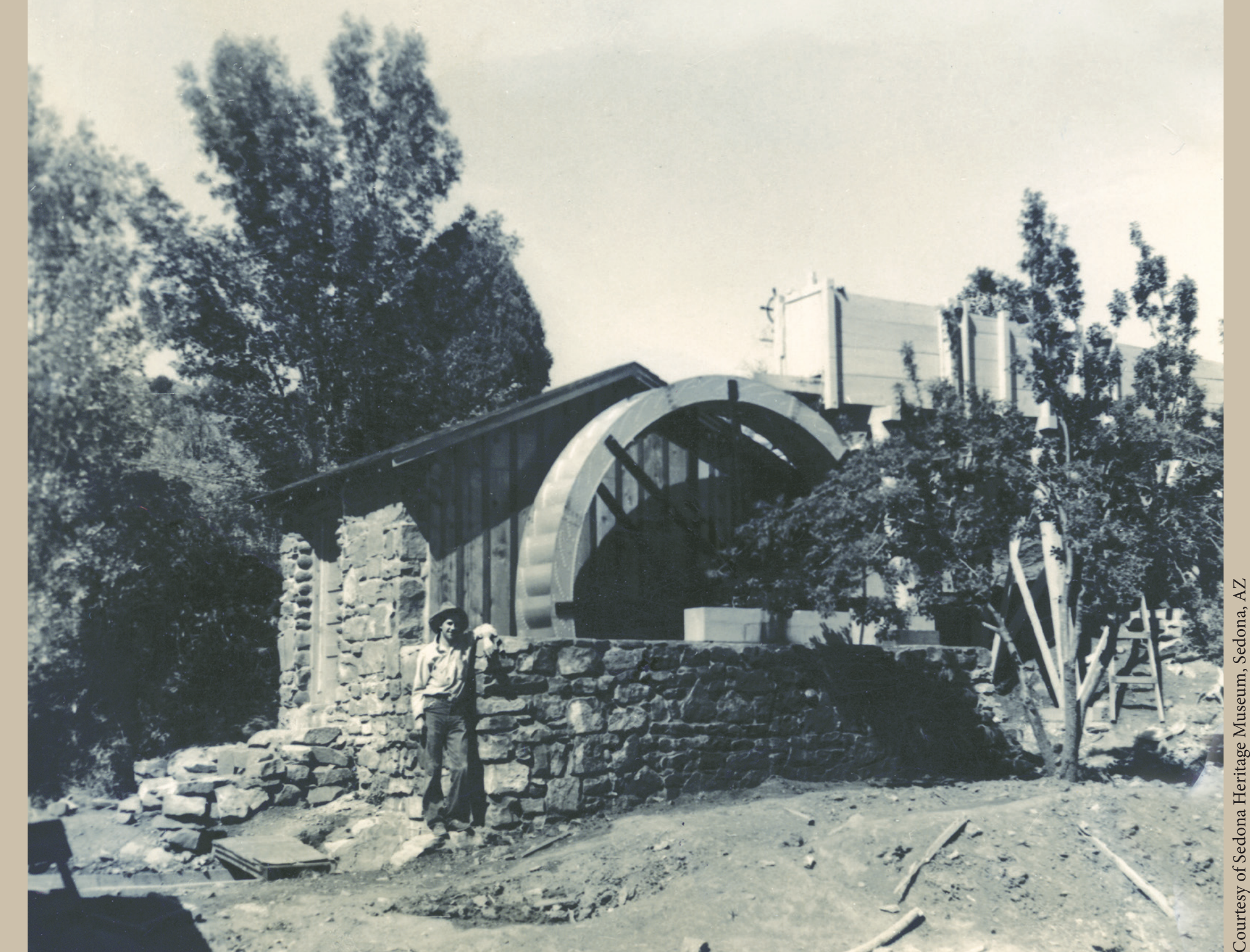
Andrew Baldwin's 14-foot water wheel (shown above) at Crescent Moon Ranch is known as an overshoot water wheel. The design, promoted by the Fitz Company, employs the force of gravity to allow water to fall from top to bottom to turn the wheel.
